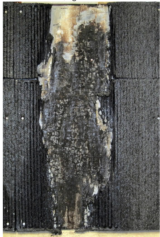
Details, right side of fire
